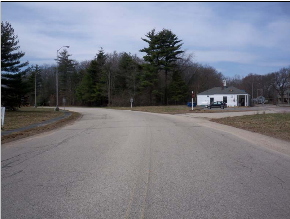
Figure A-3 Shea Memorial Drive looking west (East of Memorial Grove Avenue)
