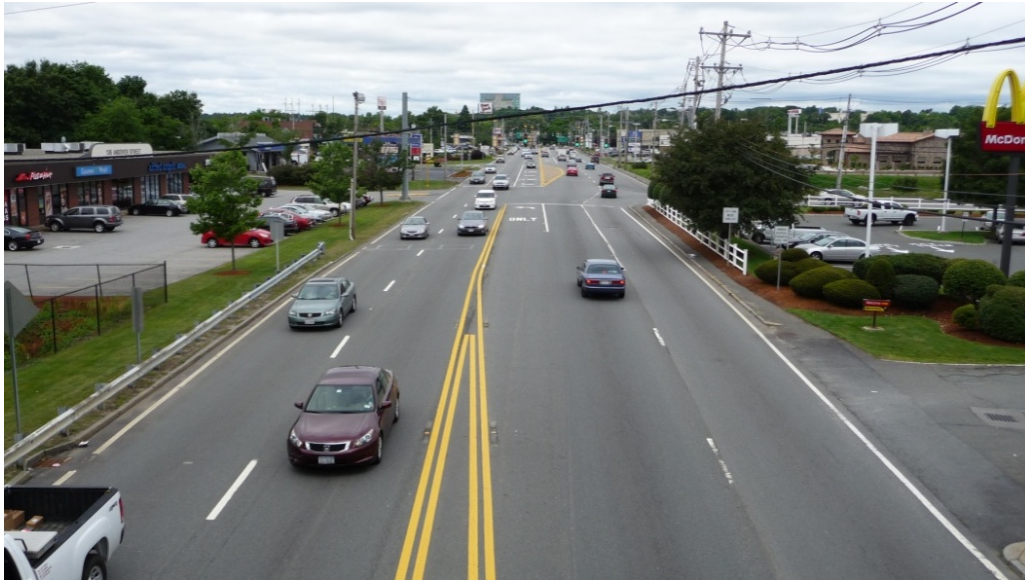
Street view, looking west from the Danvers Rail Trail bridge
