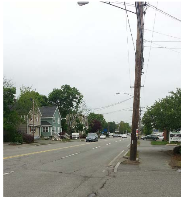
Main Street (Route 28) – Utility pole blocking vehicle and pedestrian sight lines
