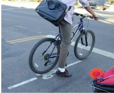
Bicycle detector pavement marking
