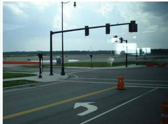
Intersection of Bill Delahunt Parkway and Shea Memorial Drive, Weymouth
